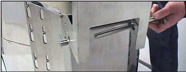
Installing the top-most rod.
